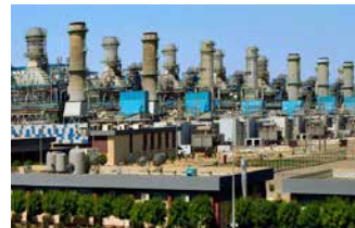
Suleymaniya Combined Cycle Power Plant - Iraq
