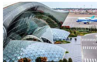
Baku International Airport Azerbaijan
